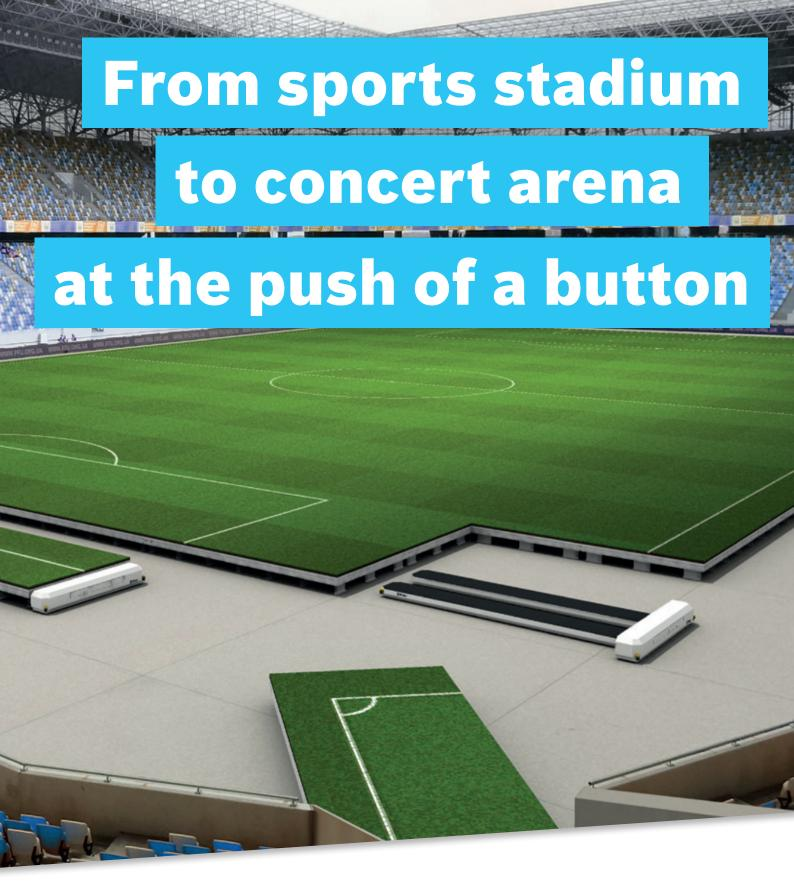
StadiaPitch is a modular and flexible alternative to other retractable pitch installations. Automated Guided Vehicles (AGV's) transport the pitch segments to a storage area either inside or outside of the stadium. This innovative and thoroughly tested solution can be integrated in existing or new stadiums. Call us now to discuss a business case for your specific situation. **We Move. You Win.**
