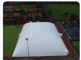
RSI double membrane installation: HOD Valkenswaard
