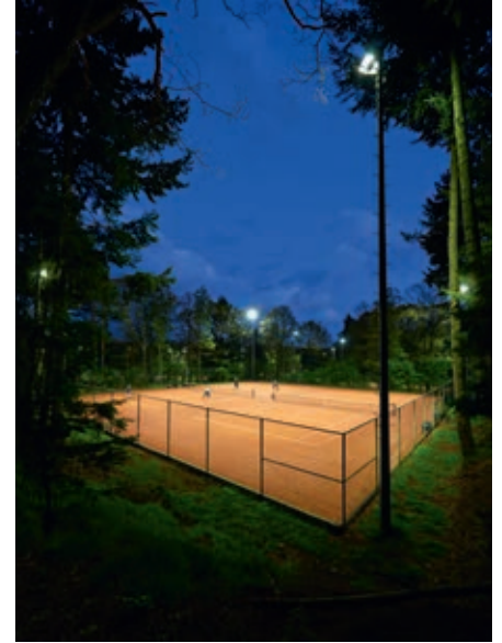
LED floodlights can be used flexibly and can achieve significant savings
